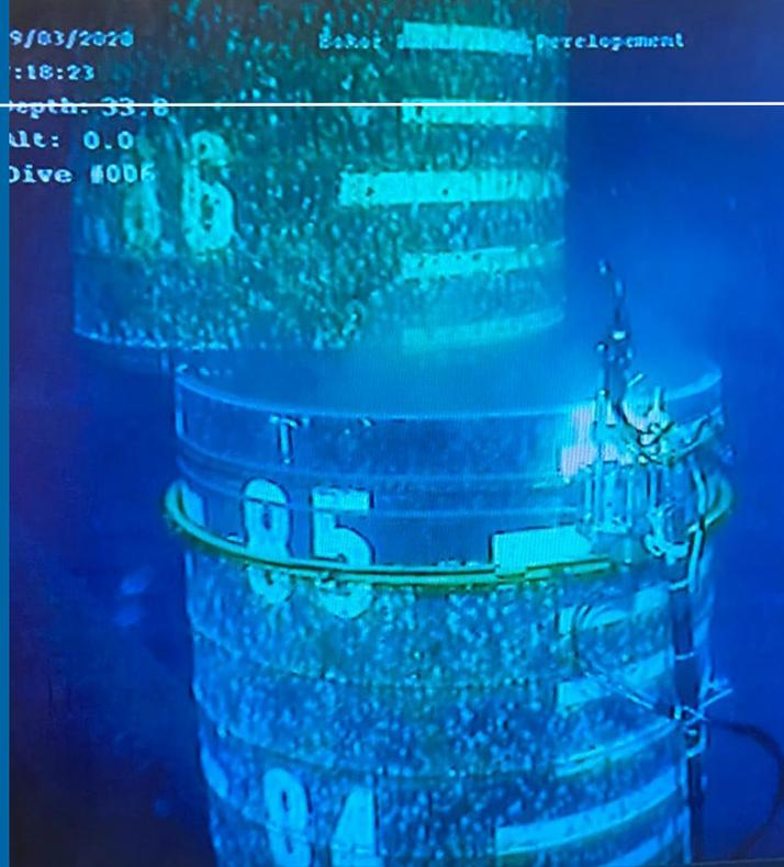
The external cutting tool was deployed subsea to the correct depth under the supervision of JFO technicians. Once at depth, divers referred to the JFO set-up procedure in order to fasten the external cutting tool to the pile.
