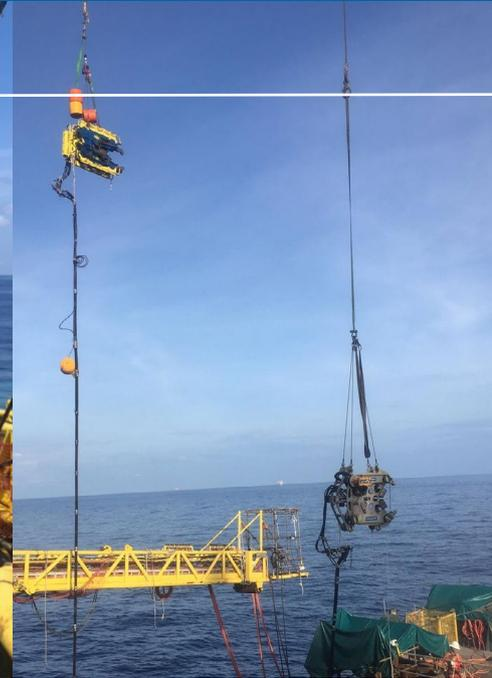
Project scope specified use of an internal cutting system with capability to cut the piles to a minimum of 5mtr below seabed level. The piles were known to contain heavy soils and these needed dredged prior to commencing cutting. Furthermore, the risers and cross member braces required to be cut externally at very specific locations, with challenging access, for optimal recovery and reef placement.
